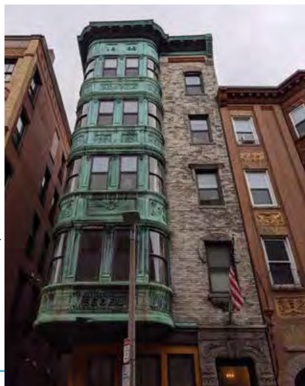
THE SEGEL BUILDING, A WHOLESALE AND RETAIL BUILDING BUILT IN 1896
